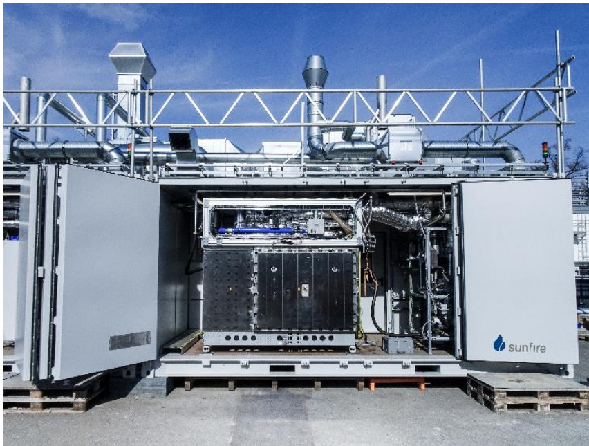
Sunfire's SOEC Module "Generation 2" (225 kW) © Sunfire GmbH
